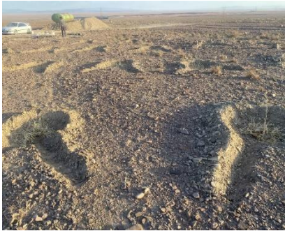
Fig 5. Construction of crescent-shaped catchment in the study area
