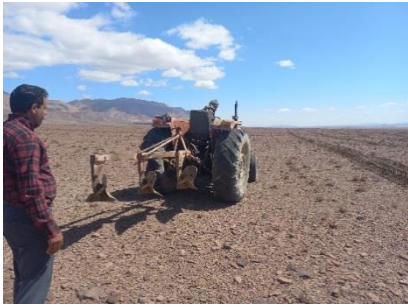
Fig 3. Bed Preparation and construction of rainwater harvesting systems
